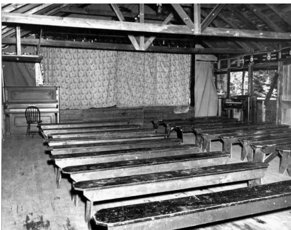
1950s Inside the Lodge
